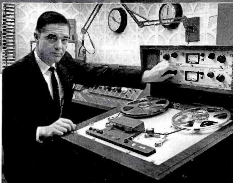
Mr. Owen checks WKRC-FM's Model 280-SP/14, Scully's 2-channel Solid State tape recorder for 14 inch reels.
